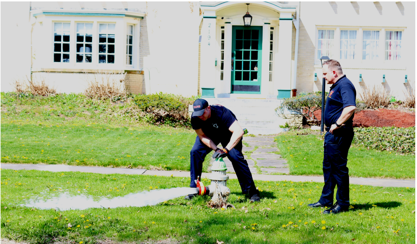
The Fire Department flushing out a fire hydrant
