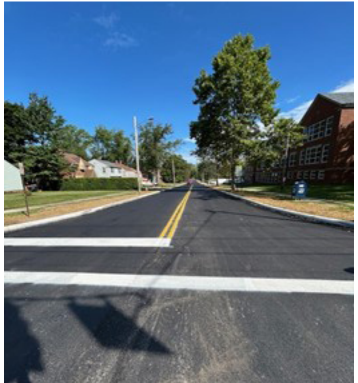
Yellowstone Reconstruction Project
