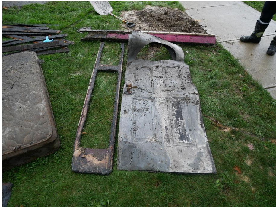
Exhibit 4: Front door located at area of origin
