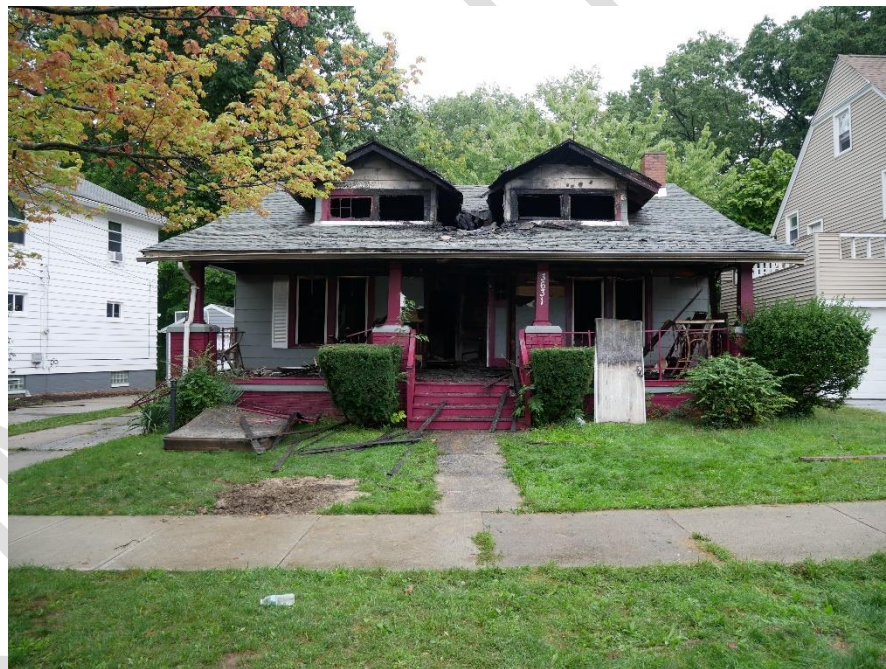
Post Incident Comparison of 3631 Randolph Rd immediately after fire.
